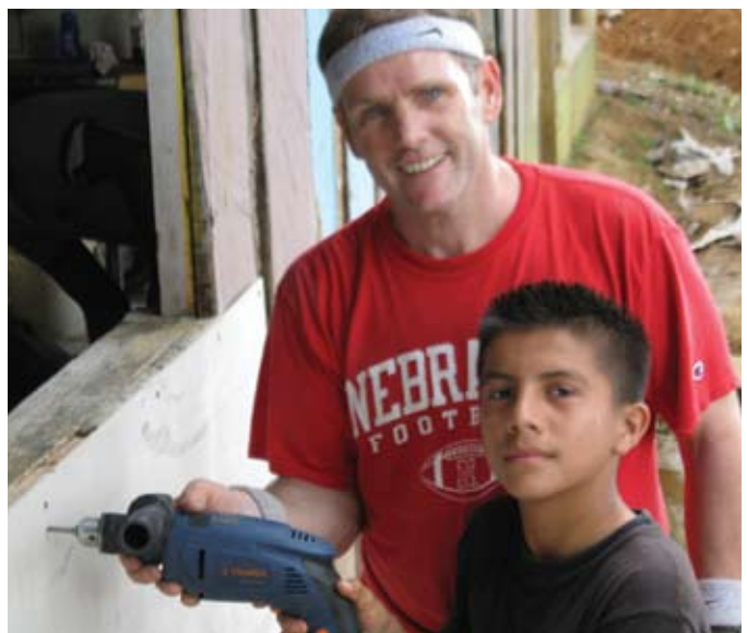
Renovation on the school – BTC volunteer teaching JGHS student to drill.
